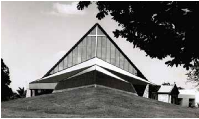
The view from Smith St. Children used to ride their bicycles up the mound and onto the roof, so we cut out the chunk at the top of the mound to prevent it, as you see it today.
